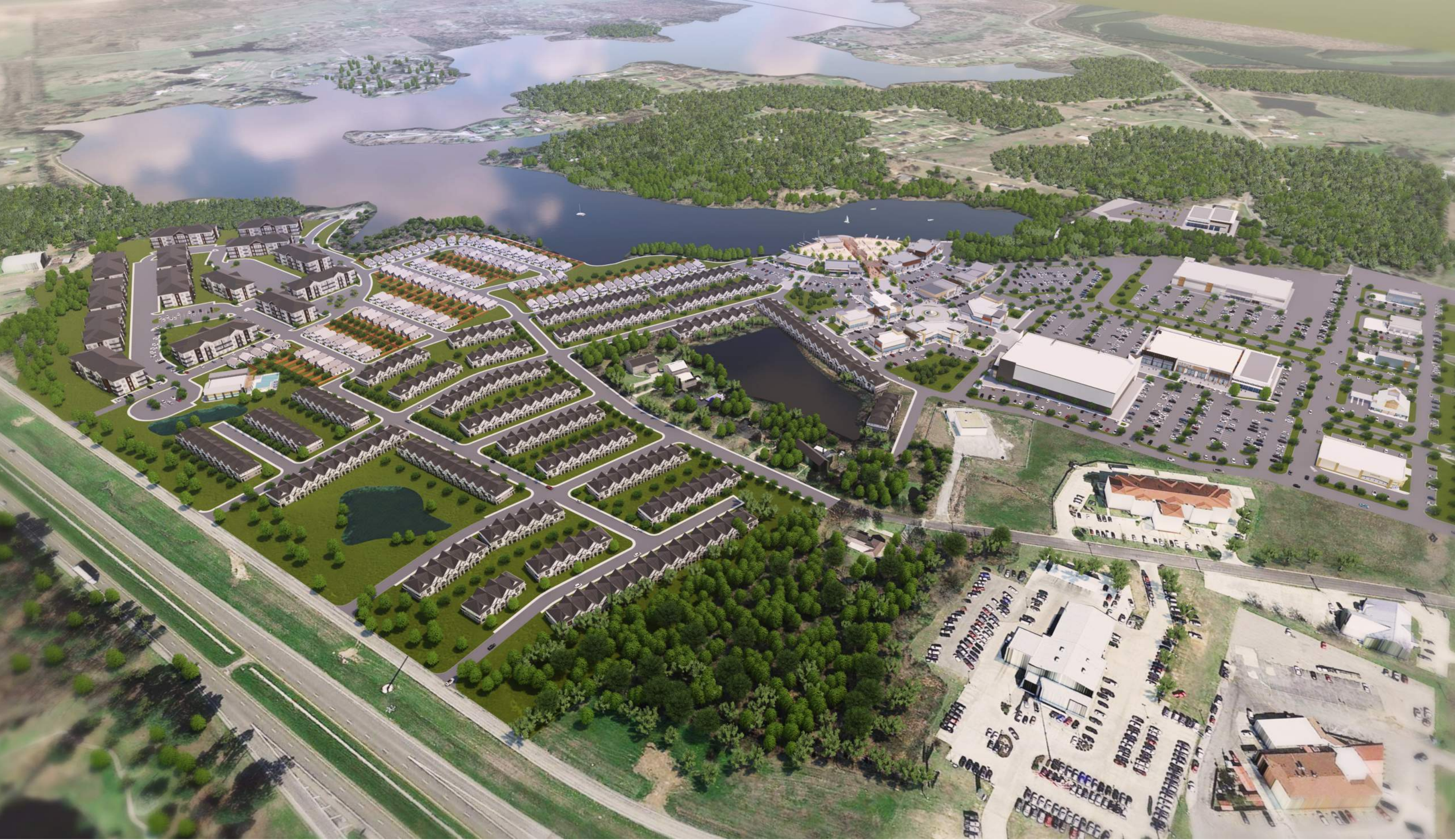
VIEW // 01 ANDERSON TOWN CENTER
